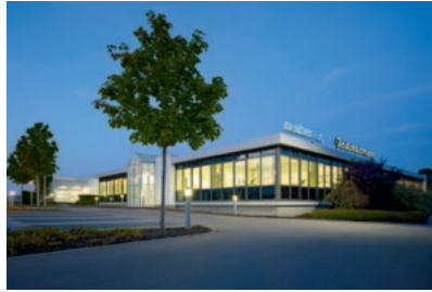
Neuberger building automation in Rothenburg o.d.T.
