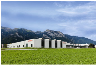
Boiler production in Sennwald
