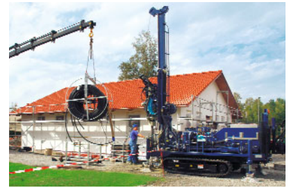
Borehole drilling by BauGrund Süd
