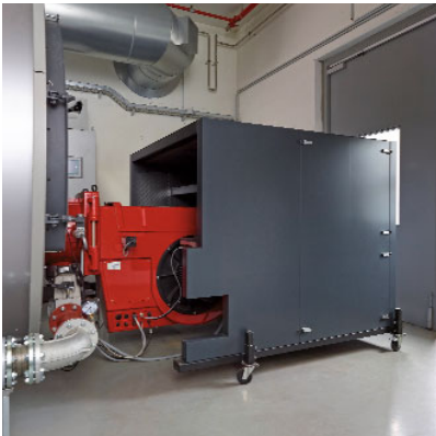
W-SH 20 in a district heating centre, with bespoke shroud cutouts for the fuel and power supplies.
