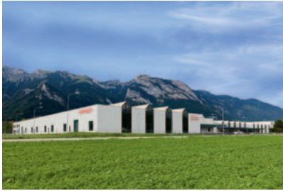
Heating system production in Sennwald
